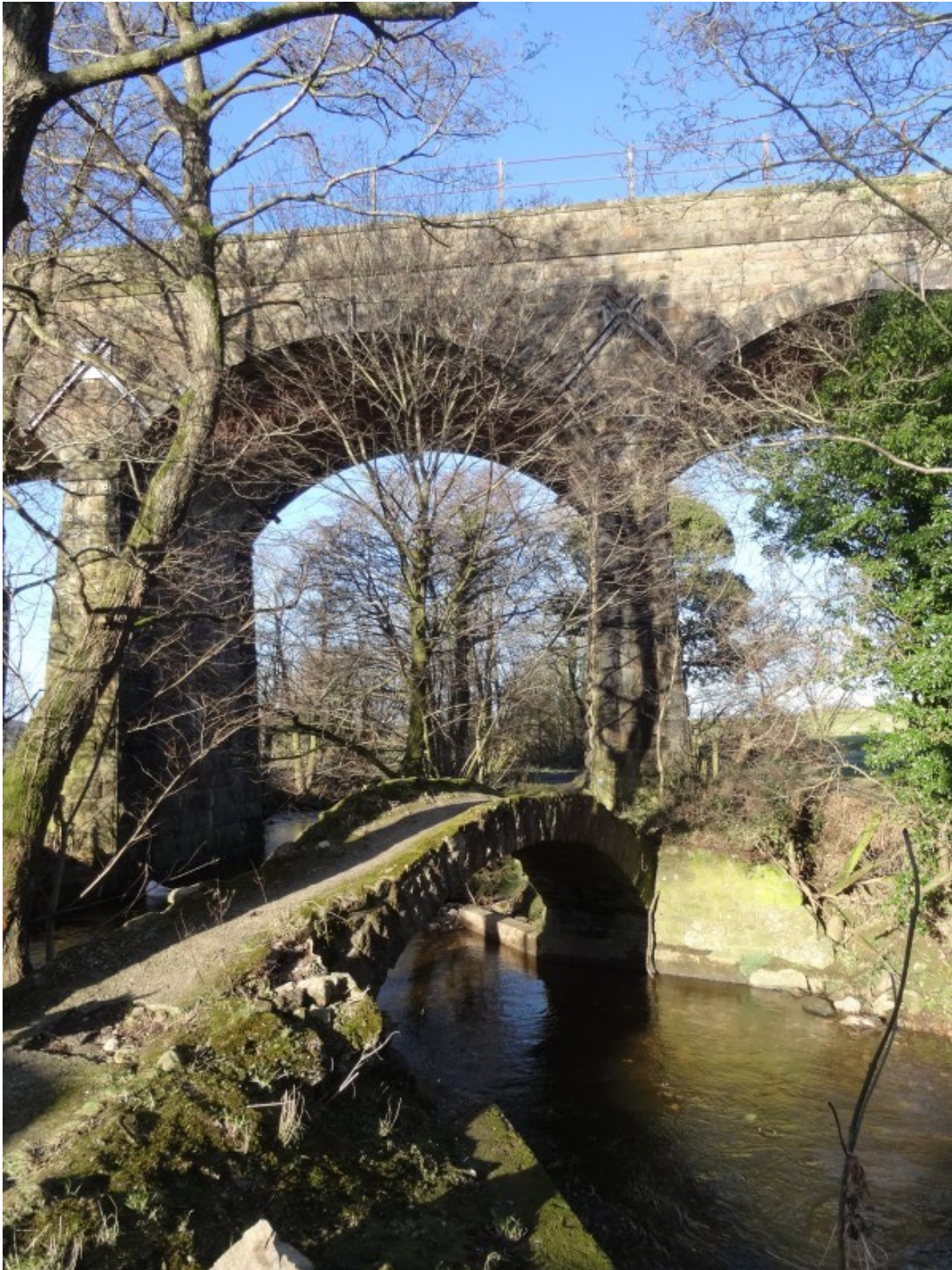
Ancient and (nearly) modern: Capernwray packhorse bridge and railway viaduct (open 1867) Peter Clinch
